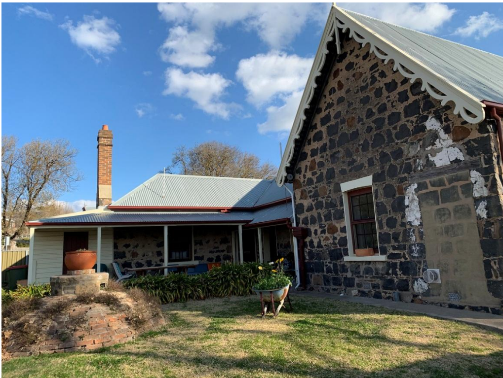
Figure 38: Block D West facade. Note filled in former doorway on right.
