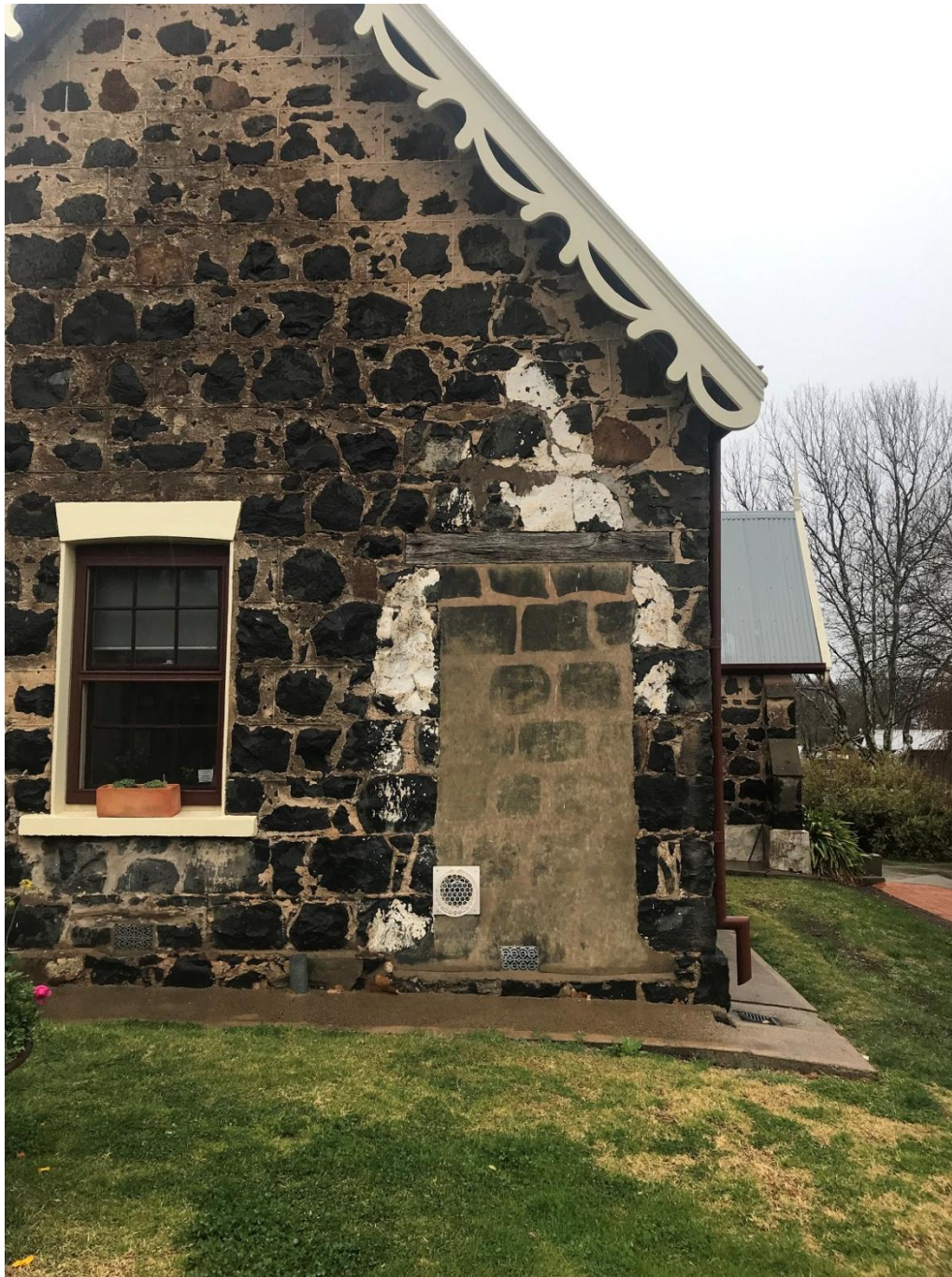
Figure 41: Detail photo of in filled former doorway. The infill is lightweight and plastered over with the apparent stonework an applied finish in paint. White paint applied to the stone wall outlines the former portico which existed here. A square hole in the concrete path at the very corner of the building is believed to be a remnant of the former fence which separated Block D when it was used as a residence from the rest of the school.
