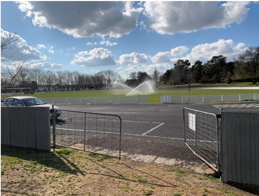
Figure 58: Along northern boundary facing the park is a grey metal panel fence with metal posts, timber rails and metal rural style gate.
