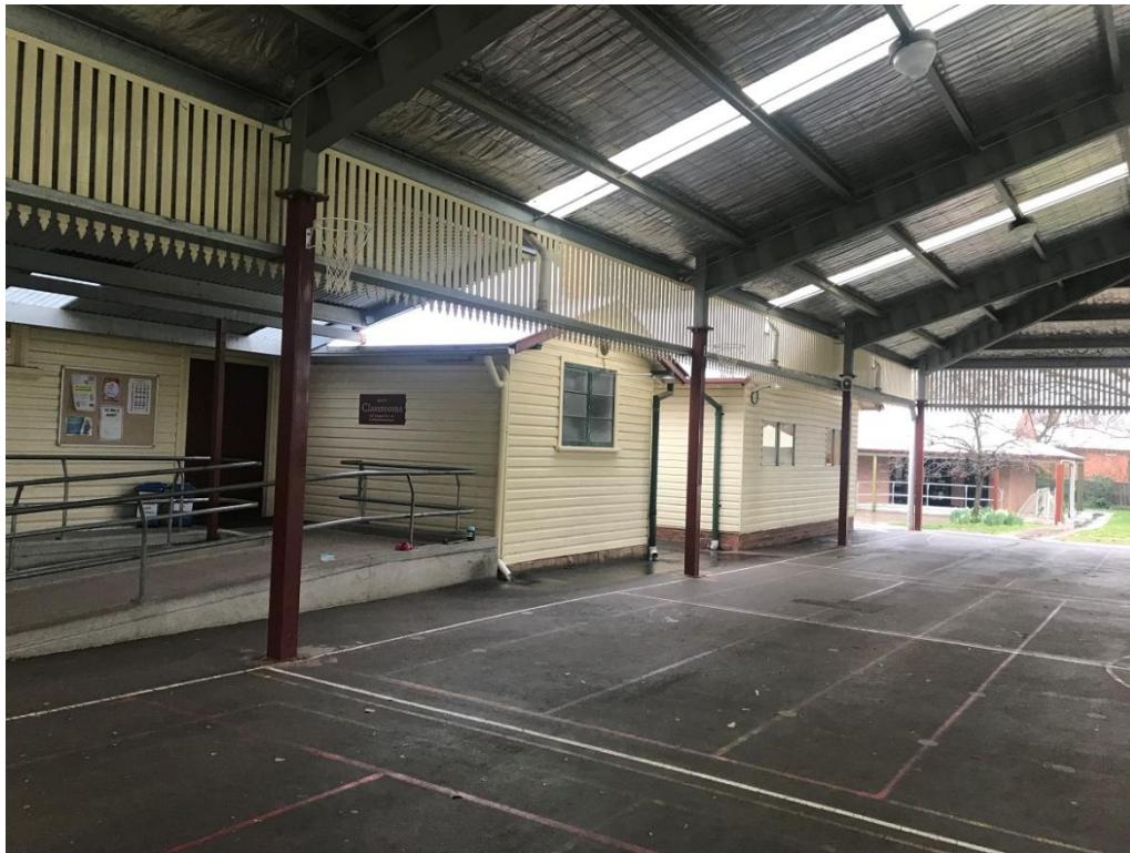
Figure 23: Block B Eastern facade with multiple additions clad in painted weatherboard.
