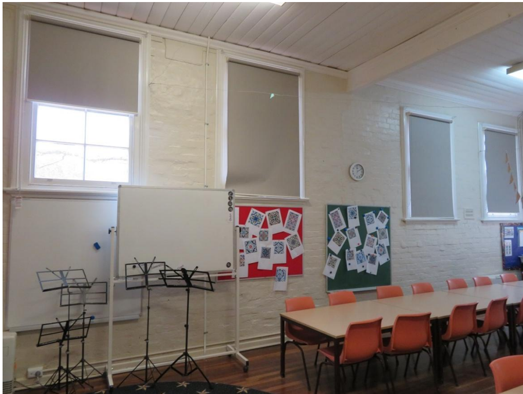
Figure 34: Block C internal view. Note the centre beam across the ceiling separating original building and addition. The window heights and direction of ceiling cladding change either side of the beam.
