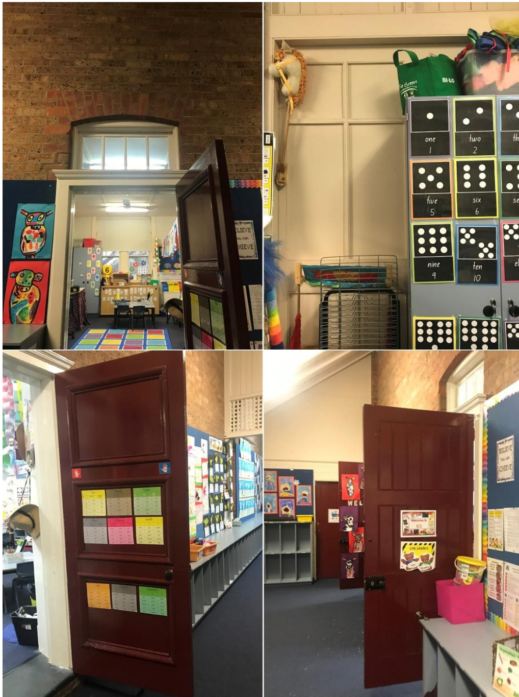
Figure 31: Block B internal details - clockwise from upper left. Door heads with high-lites between verandah and classrooms. Glazed partitions between classrooms which have been painted over. Classroom door panels front and back.
