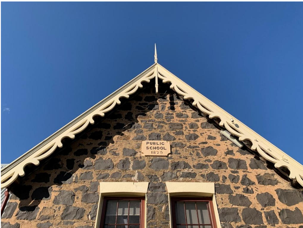
Figure 36: Detail photo of gable, bargeboards, pendant and finial, window heads and building plaque.
