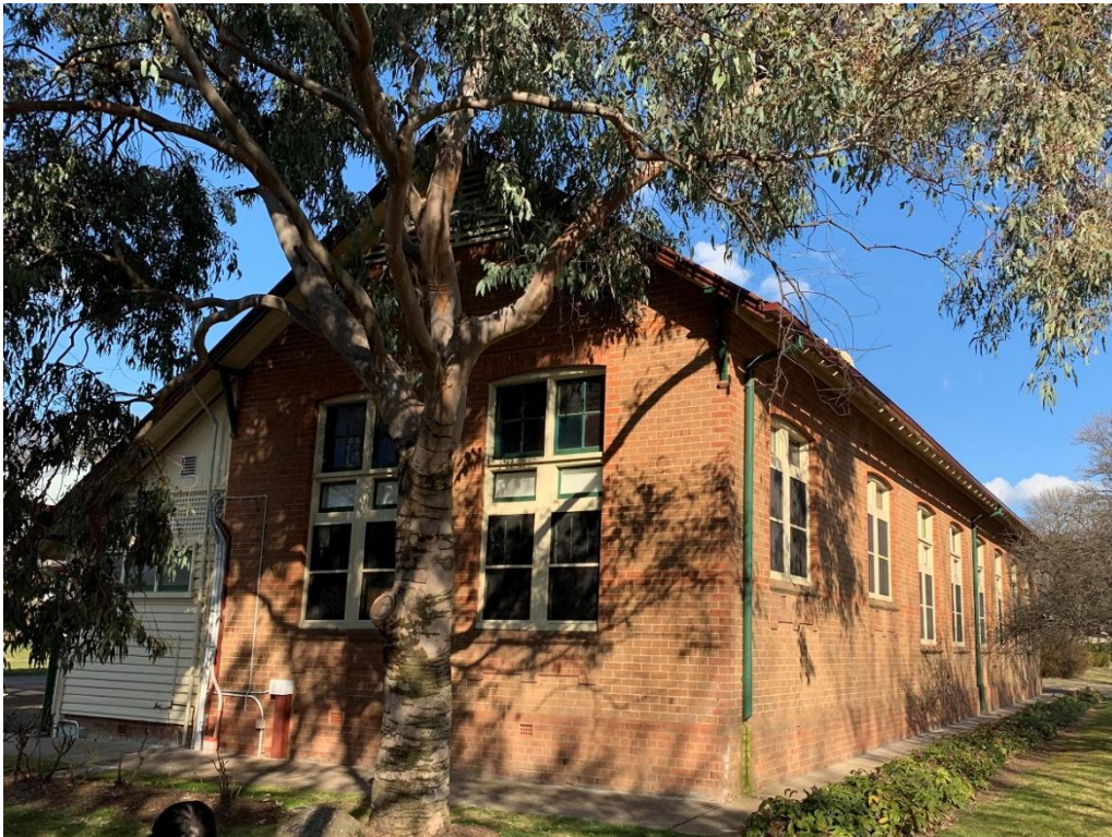
Figure 26: Block B north and West facades. Note the difference in sill height of the northernmost windows on the west side. This is the original configuration of the typical windows. The larger windows date from design of the 1911 alterations.
