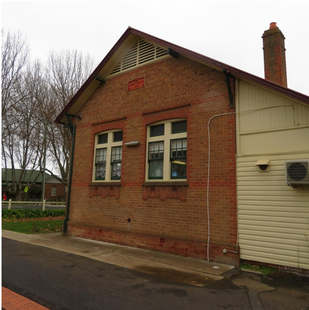
Figure 21: Block B southern facade showing the original configuration of design details e.g. window sizes, head and sill details, vented gables, eaves linings and brackets etc.
