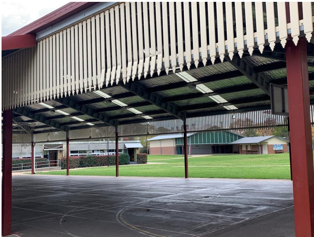
Figure 53: Shade structure looking northeast toward Hall. Note bent pickets to frieze.
