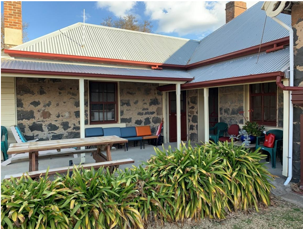
Figure 39: Detail of former residence portion of Block D. Note clashing verandah roof lines in the corner suggesting alterations.
