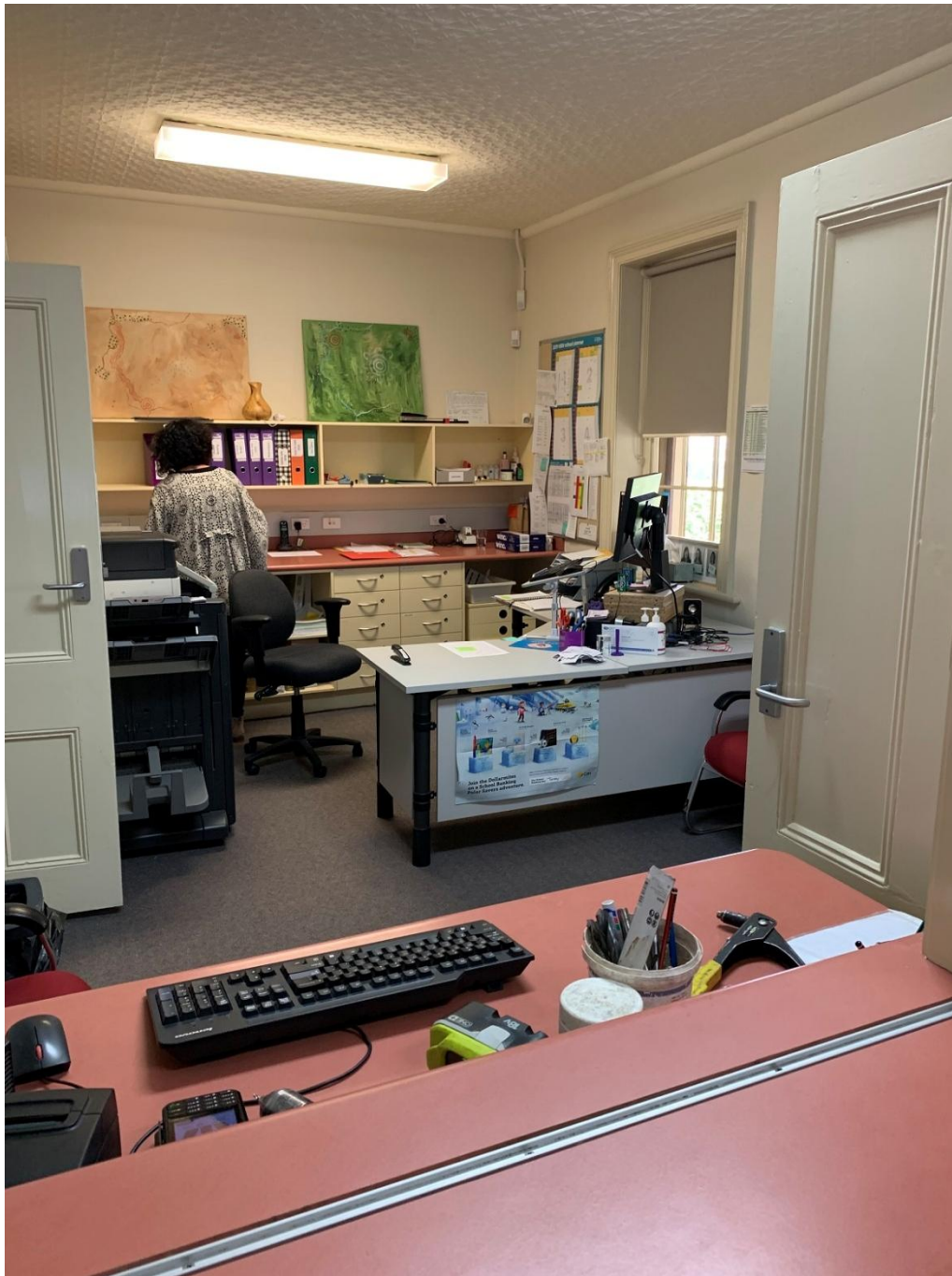
Figure 43: Inside the admin office in Block D. Door panels and architraves may be original though door hardware is clearly not. The pressed metal ceiling is expected to be an alteration circa the 1890s to early 20th century.
