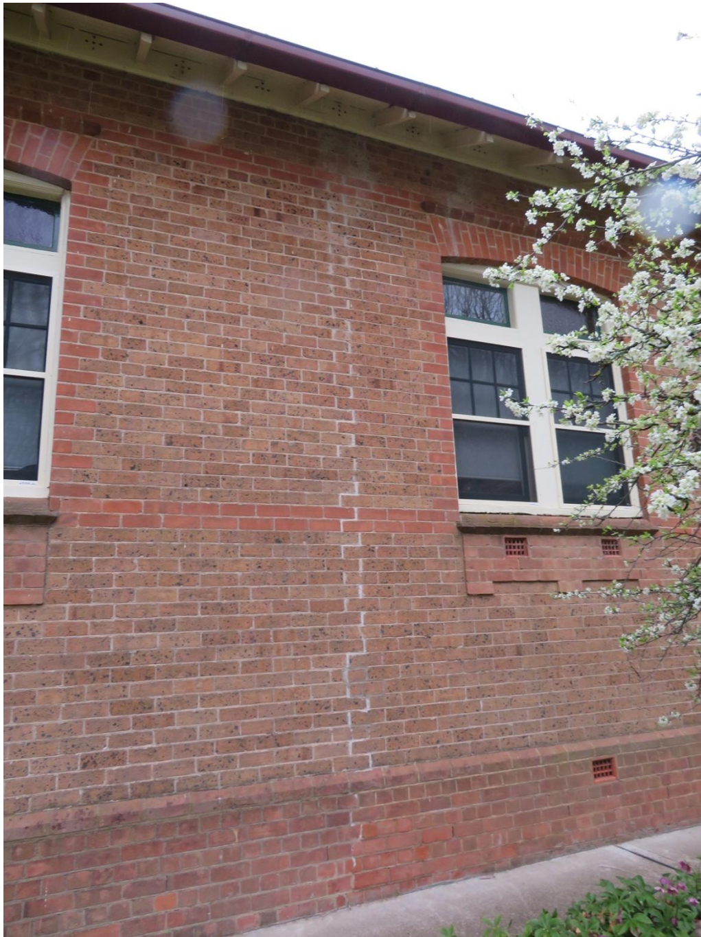
Figure 27: brick joint where the 1911 additions were keyed into the earlier structure.
